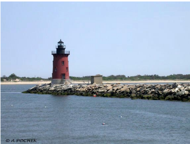
Delaware Breakwater, DE
