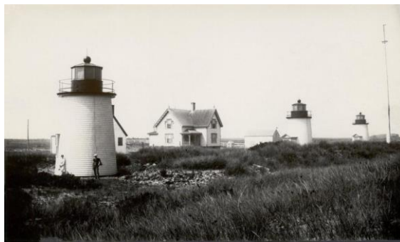
Wooden towers replaced the brick ones in 1892
