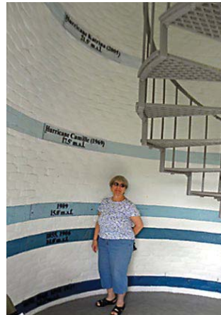
High water marks with Hurricane Katrina at the top at 21½ feet..
