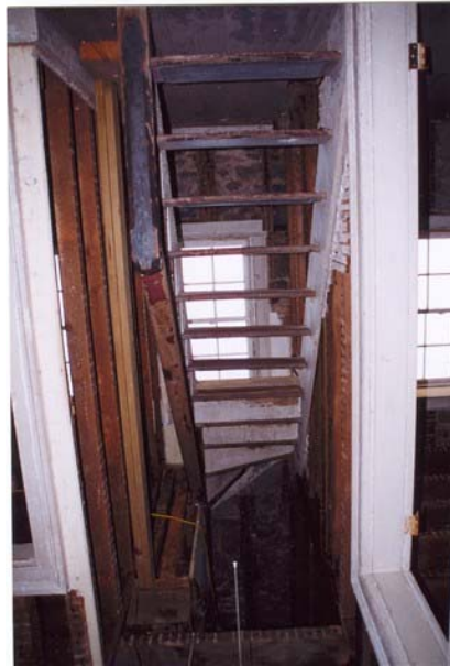
North Light, BI -- Stairs to be replaced with NELL Grant
