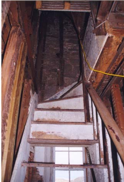
North Light, Block Island - Stairs to be replaced with NELL Grant
