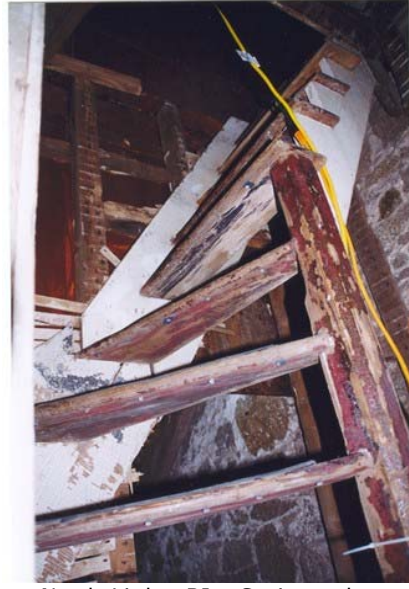
North Light, BI - Stairs to be replaced with NELL Grant
