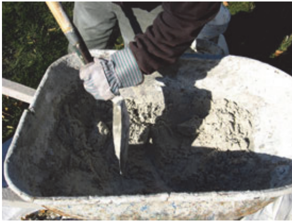
A close-up view of the cement mixture being prepared for application
