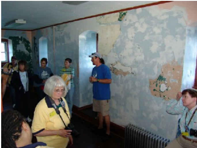
The walls of one of the rooms undergoing restoration
