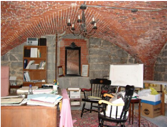
Arched brick ceilings and granite walls in 1st basement in Custom House
