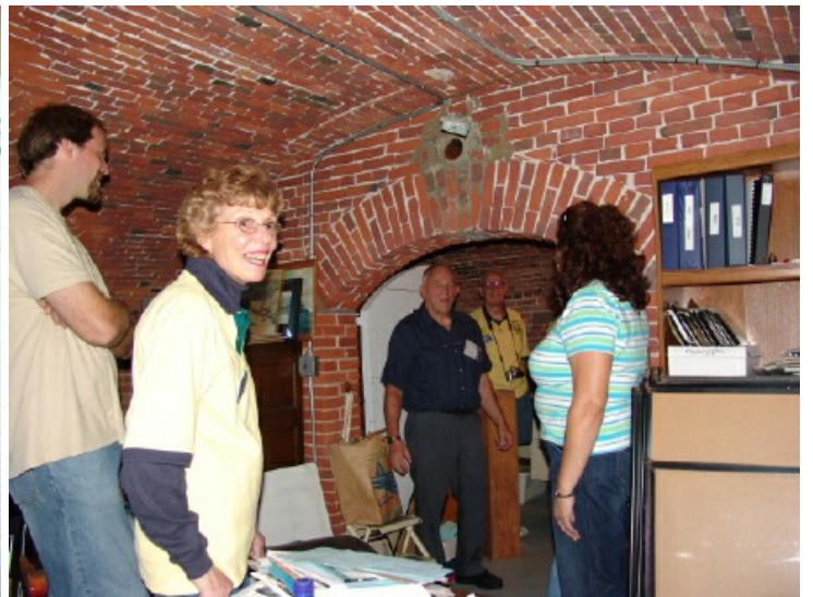
1st Basement in Custom House has arched brick ceilings
