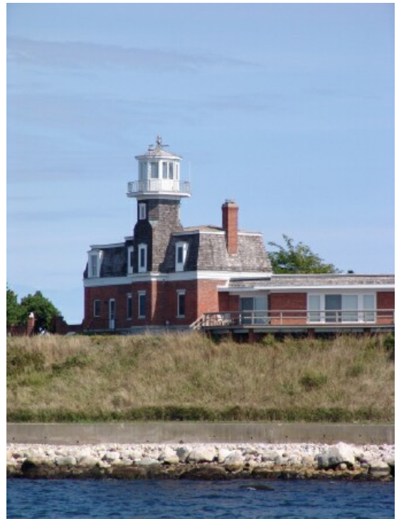
North Dumpling Island lighthouse
