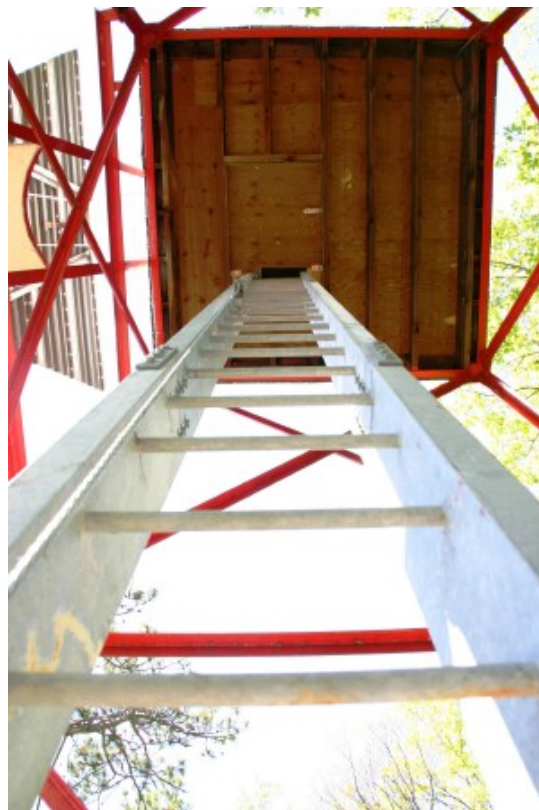
Ladder and entry hatch of DeWatteville Rear Range
