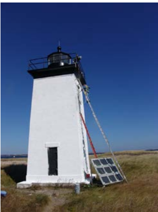
Nice paint job so far
