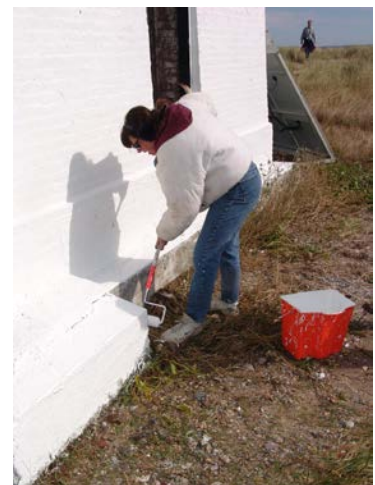
Lynne Kerber finishes around base
