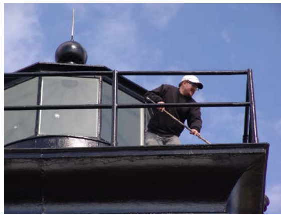
Bob uses a roller to paint parapet black
