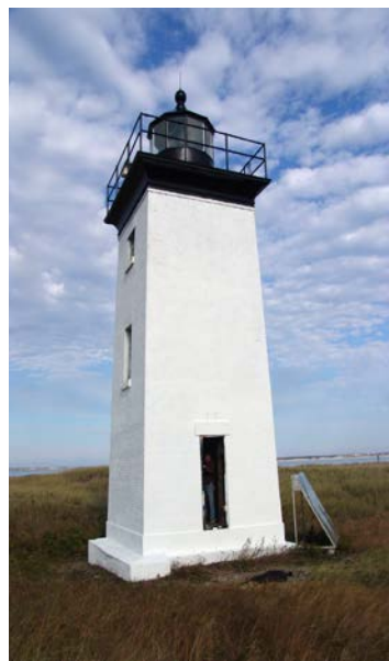
A completed tower stands proud with a new paint job.
