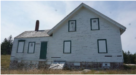
Left side of the Keeper's House
